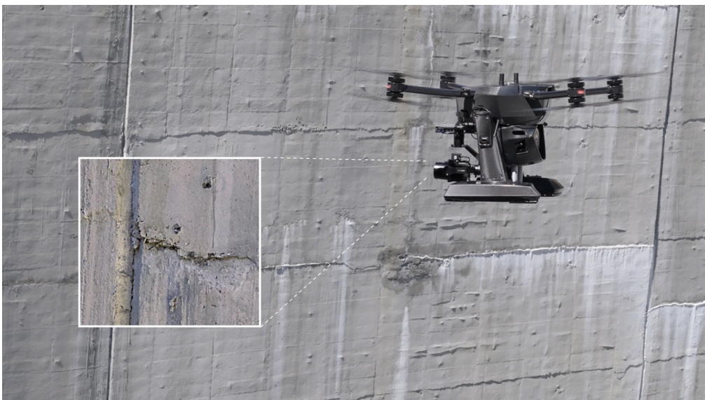
Photo: High-resolution dam inspection using the Xer X8 UAS and Phase One P3
